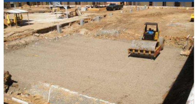
Rafael Cordero School, Cataño
